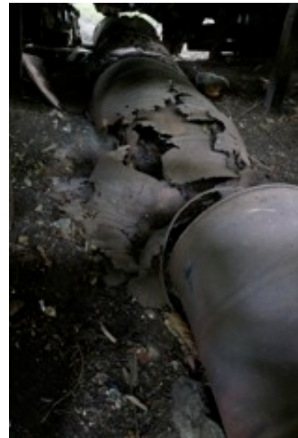
Photo 6. Broken oven tunnel of a locally built oven made of barrels
